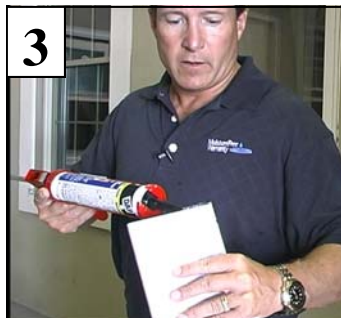
3 Apply sealant along the edge that will be placed against the jamb.
