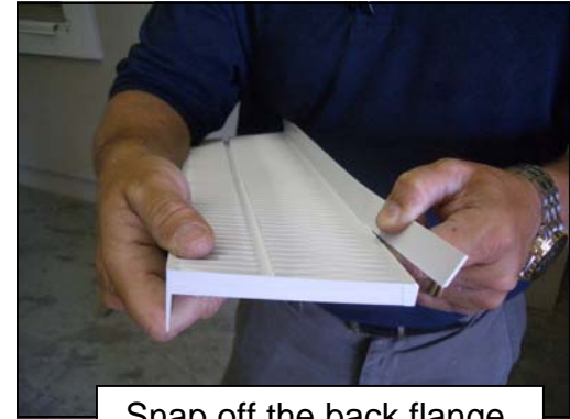
Snap off the back flange.
