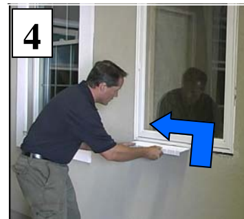
4 Push in first, then over to place caulk against jamb.
